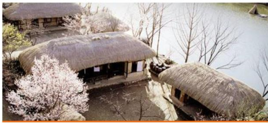
↑ Joseon Period Houses and Traditional Work Shop
